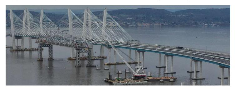
As previously reported, in September 2018, Tappan Zee Constructors (TZC), with project engineers, learned that the old Tappan Zee Bridge's east anchor span, which was already out of service, was damaged but stable with certain key components highly stressed.
