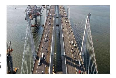
The \$3.98 billion Governor Mario M. Cuomo Bridge is one of the largest single design-build contracts for a bridge project in the United States. Located less than 20 miles north of New York City, the cable-stayed span crosses one of the widest parts of the river and is the largest bridge in New York State history.
