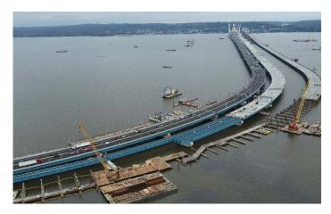
Dismantling operations began at the Rockland and Westchester landings in October 2017, after all traffic was transferred to the first span of the new Governor Mario M. Cuomo Bridge. Noise abatement measures, including temporary noise barriers, were implemented. TZC continues to monitor noise and vibration levels as work continues.
