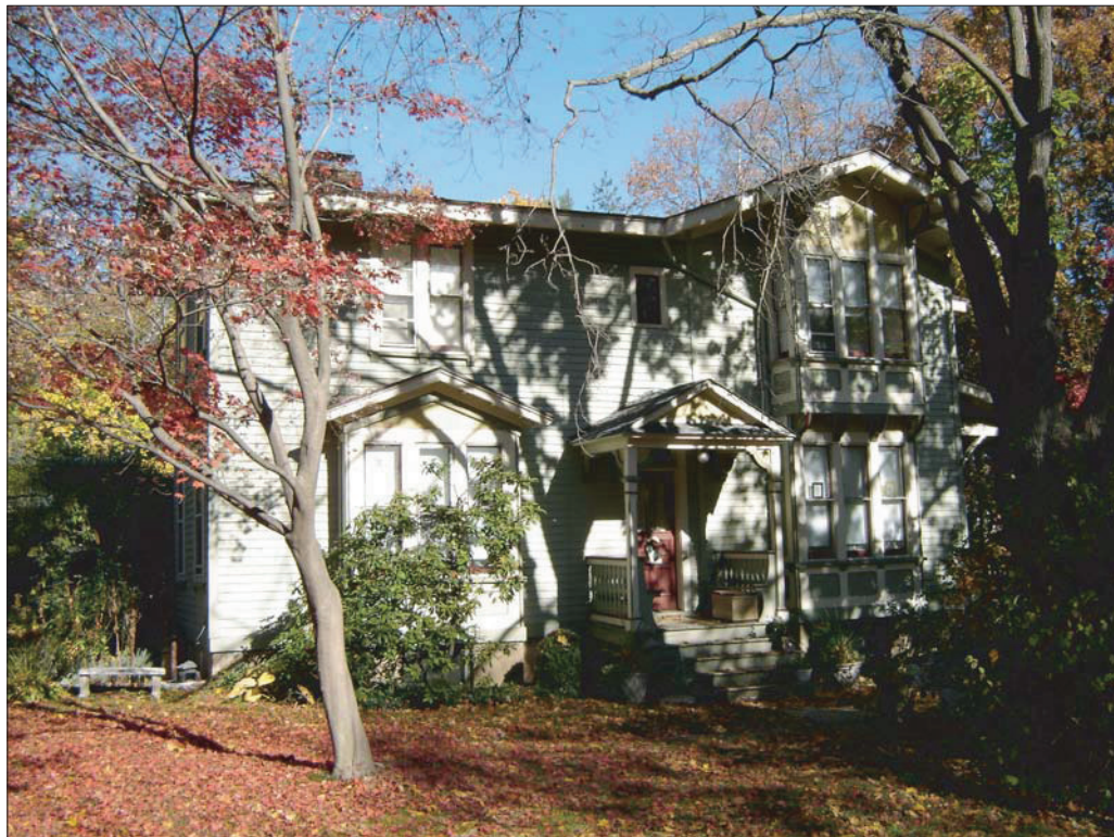
Photo 2. Looking toward south façade of 10 Ferris Lane. Note central glass-and-panel door sheltered by pedimented portico on first story. Note historic windows in wood surrounds, including gable-front bays with triple windows and diamond-pane casement window on second story.
