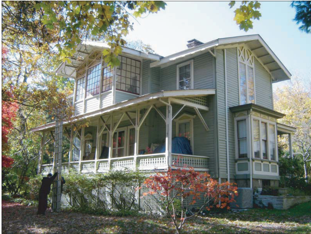
Photo 1. Looking toward east and north façades of 10 Ferris Lane. Note porch supported by wood posts with bracing on first story and central gable-front dormer with multi-pane window panels on second story of east façade. Note bay window with decorative details and gable-end embellishment on north façade.
