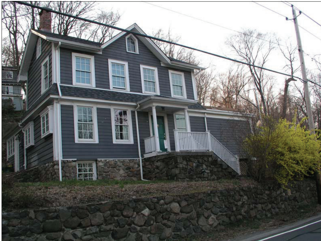
Photo 1. Looking toward east façade of 2 Shadyside Avenue. Note Gothic details including centered gable with multi-pane pointed casement window on east façade. Note historic projecting casement windows on first story of south façade.
