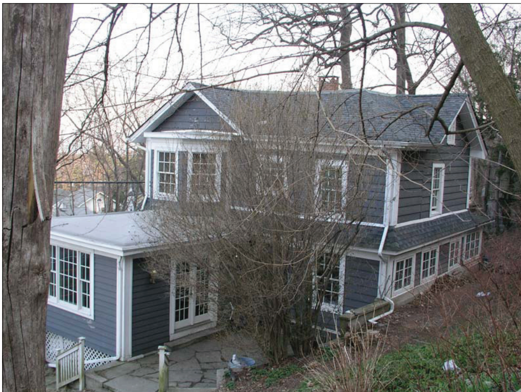
Photo 2. Looking toward south and west façades of 2 Shadyside Avenue. Note oriel window on second story of south façade. Note casement windows on first story and shuttered pointed window on second story of west façade
