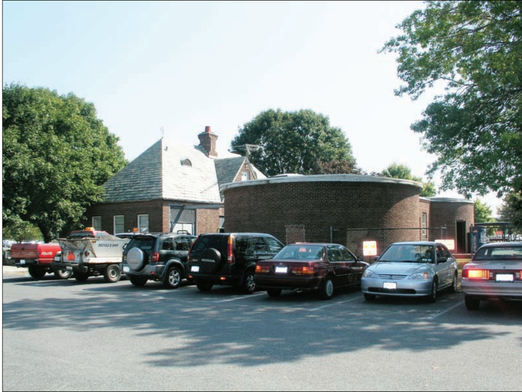
Photo 3. Looking toward north and west facades of the former Administration Building and Digester. Although building has been converted to function as an office, it retains integrity.
