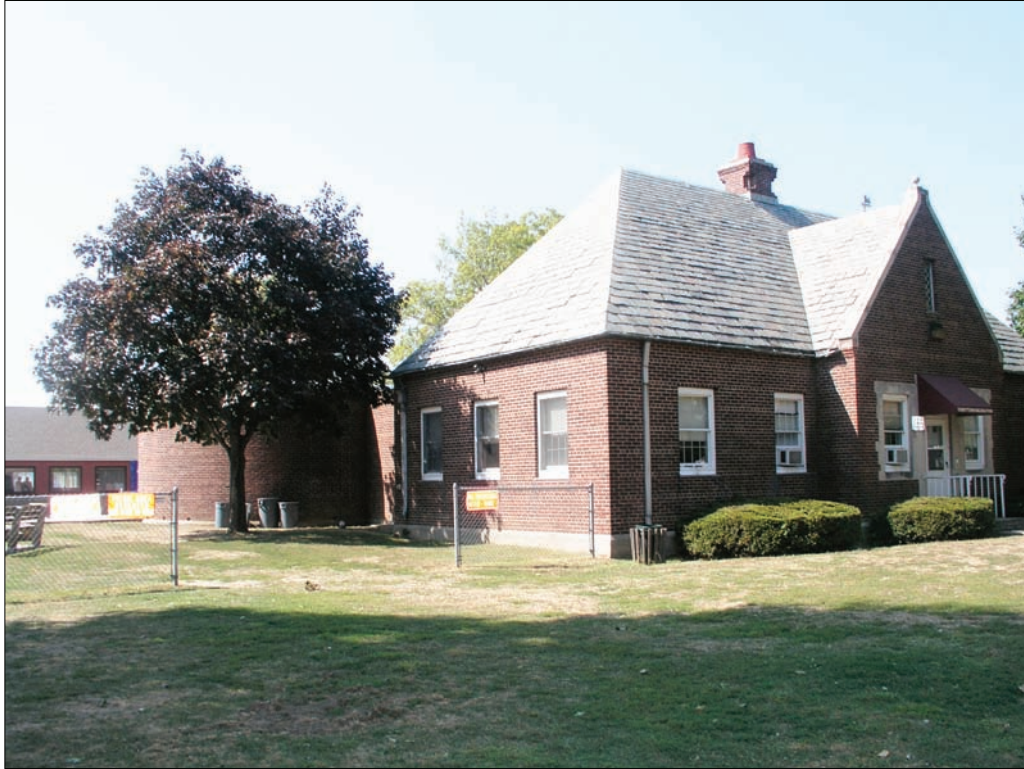
Photo 1. Looking toward east and south facades of the former Tarrytown Sewage Treatment Plant Administration Building. Note cylindrical Digester appended to the west façade.
