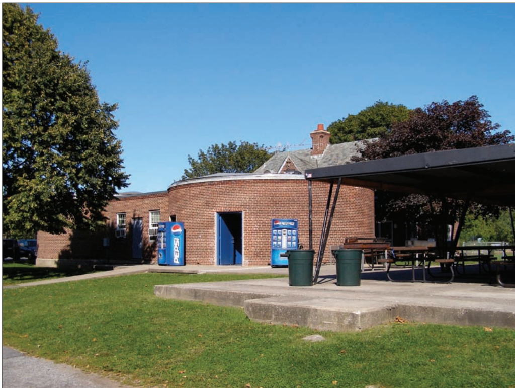
Photo 4. Looking toward west façade of the former Digester and Administration Building.
