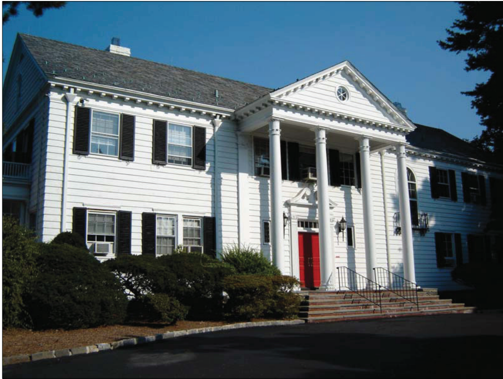
Photo 1. Looking toward main, or west façade of 100 White Plains Road. Note full-height Classical-style entry portico; principal entry set within broken-pediment door surround; and historic fenestration.
