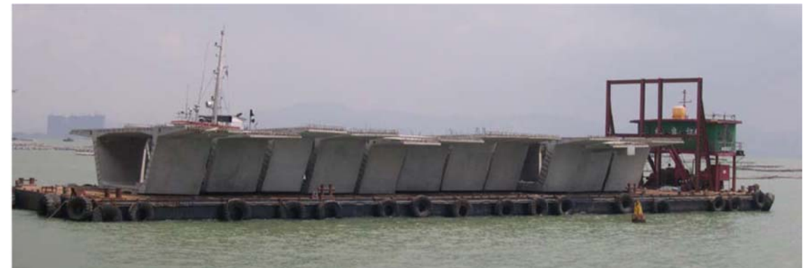
Figure 6.2 - Delivery of cast segments on barges
