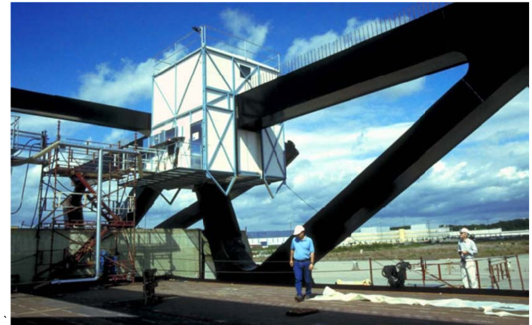
Figure 6.8 - Fabrication Yard – welding enclosure
