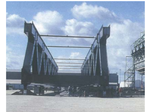
Figure 6.10 - Fabricated Truss Unit
