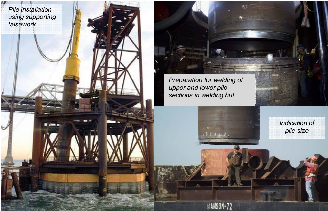
Figure 5.7 - Pile Installation
