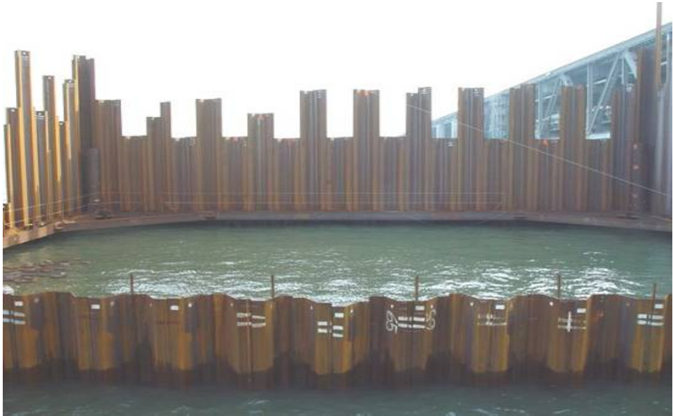
Figure 5.1 - Standard Cofferdam
