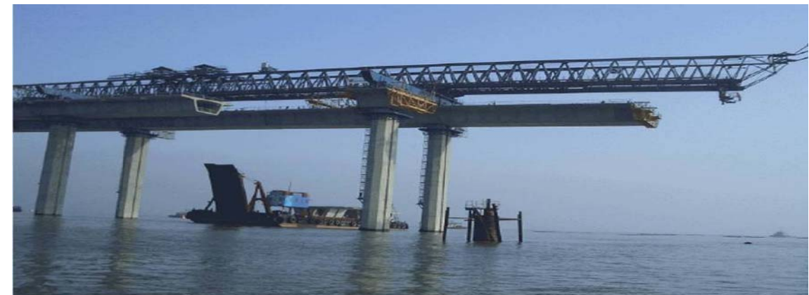
Figure 6.3 - Overhead gantry installs segments
