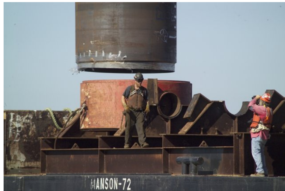
Figure 4.14 - 10 foot Diameter Steel Pile as used on the San Francisco Oakland Bay Bridge
