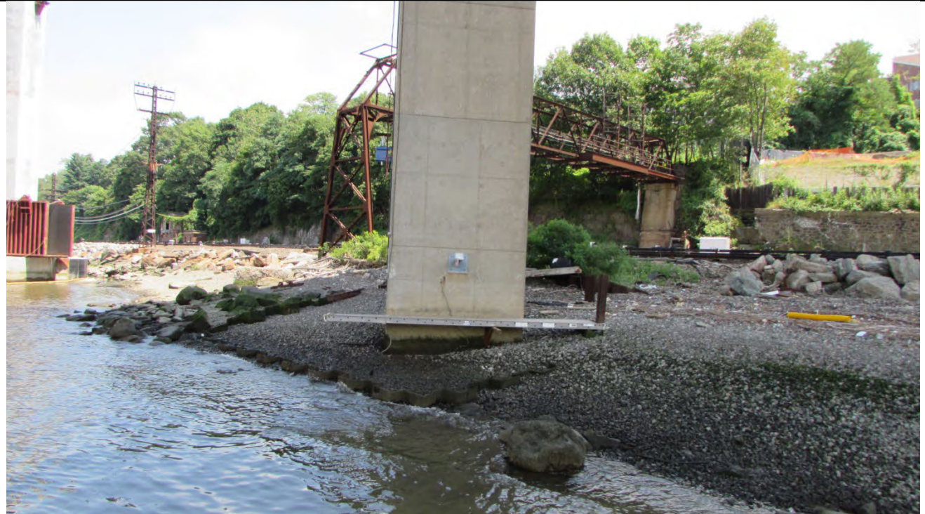
Figure 3 – Northern Pier Bent 190 at Low water, July 27, 2015, looking northeast. The remains of a sheetpile cofferdam which surrounds the pier bent.
