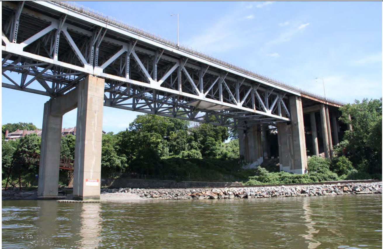
Figure 1 –Pier Bent 190 and 191 at Low water, August 15, 2013, looking northeast. Pier Bent 191 is on the right hand side where the underdeck truss terminates.
