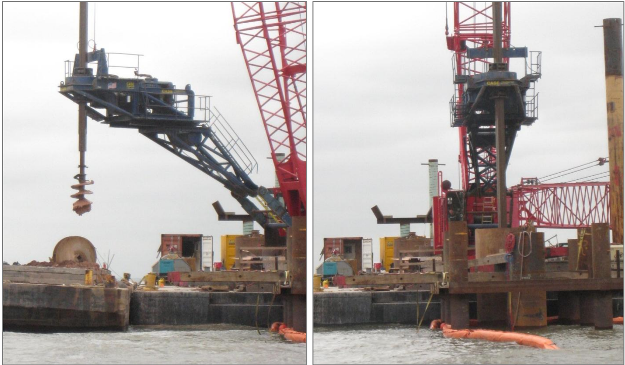
Figure 17. (Left) 60-inch auger bit at Test Pile 3B, 12 June 2012. (Right) Drill inside casing of Test Pile 3B.
