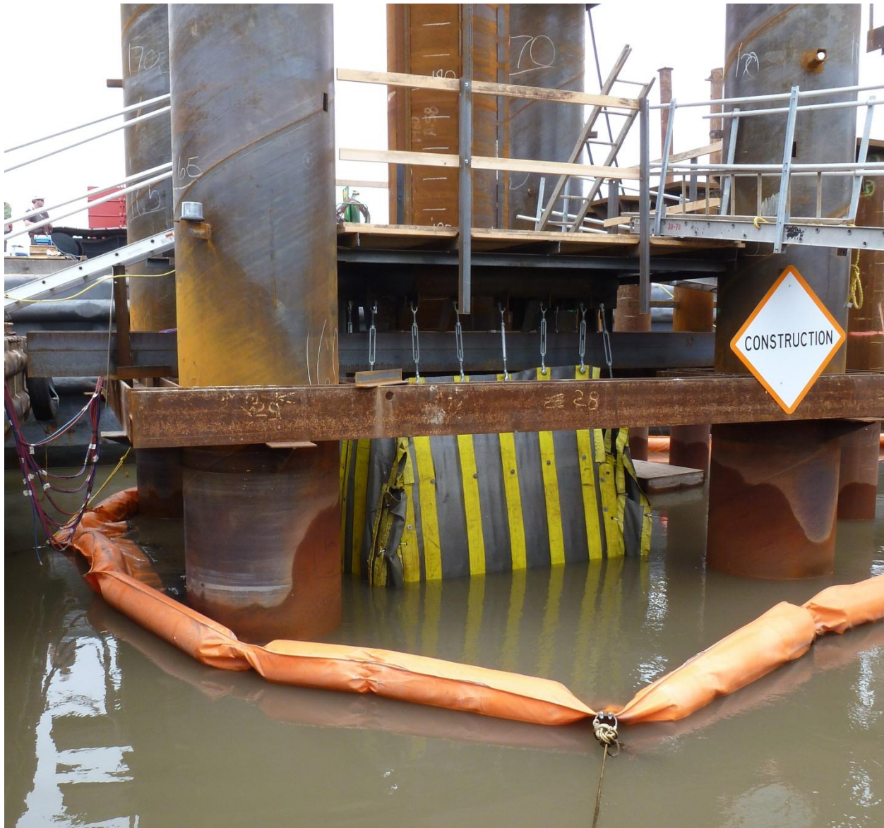
Figure 5. Photo of the base of Test Pile 1B showing the containment curtain for the Hard Bubble Noise Attenuation System (yellow and gray) and the turbidity curtain top floats (orange).
