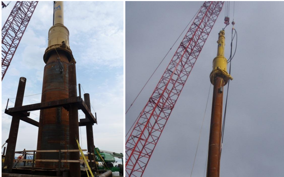
Figure 3. (Left) MENCK MHU 800S hydraulic impact hammer being lowered onto Test Pile 4A on 14 May 2012. (Right) MENCK MHU 270T hydraulic impact hammer being lowered onto Test Pile 1A on 5 May 2012.
