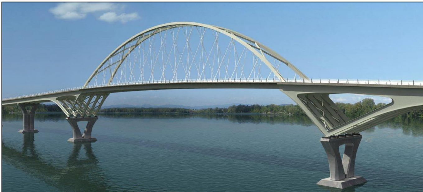
Example of Arch Option (Lake Champlain Bridge, New York/Vermont)
