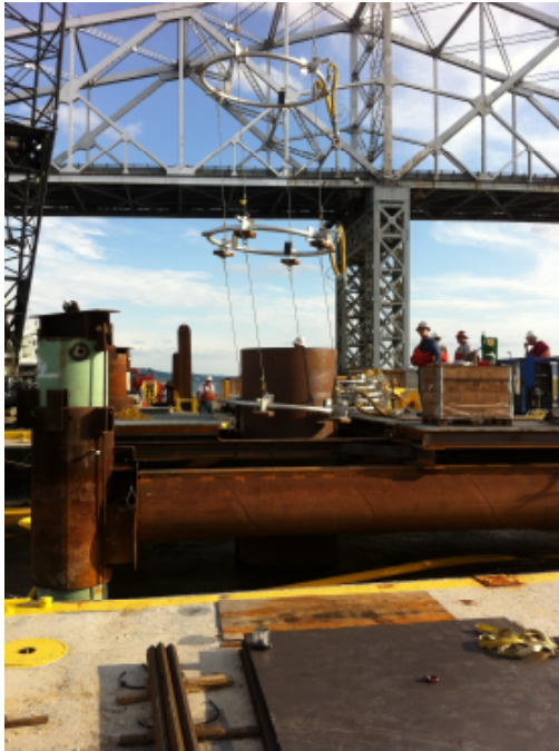
Figure 3. Deployment of the Unconfined Multi-tier Bubble Curtain
