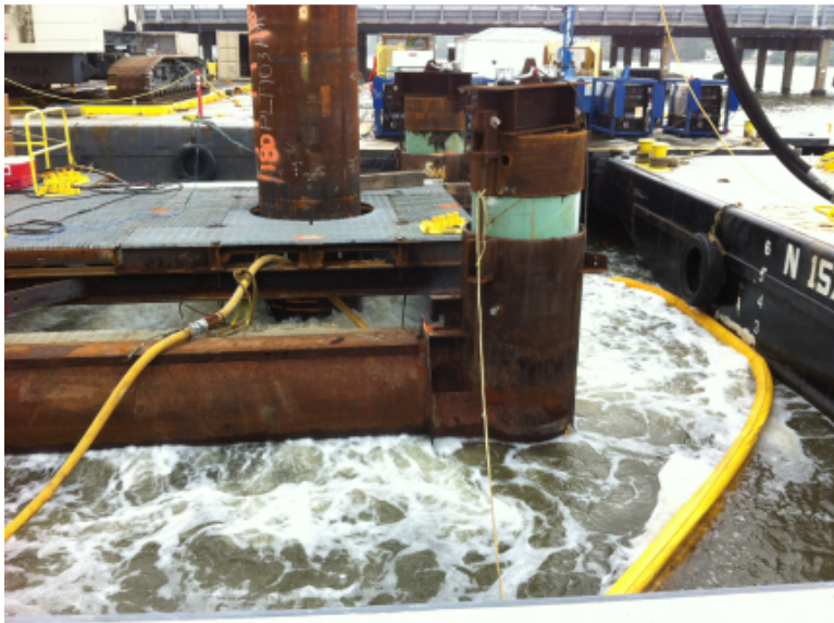
Figure 4. Operation of the Multi-tier Bubble Curtain
