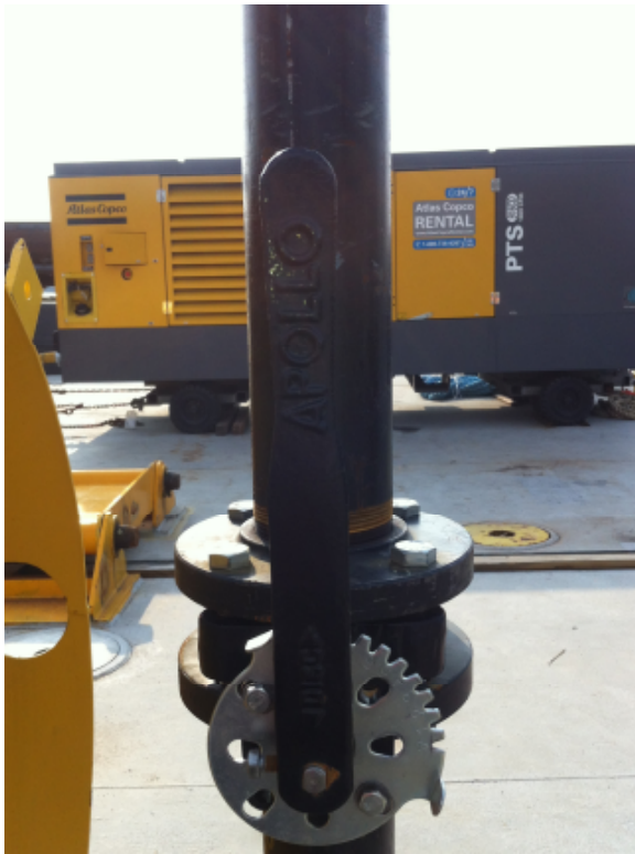
Figure 8. Valve at the Outlet from the Reservoir Tank to the Bubble Curtain
