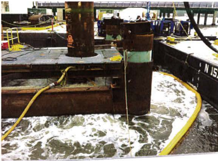
Figure 4. Operation of the Multi-Tier Bubble Curtain (One Ring Deployed)
