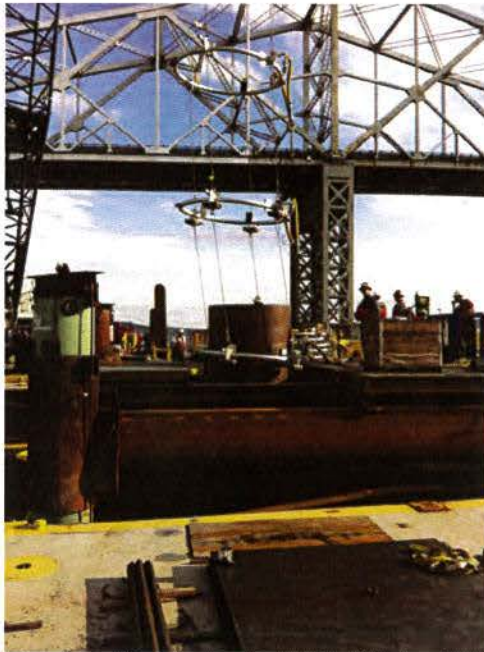
Figure 3. Deployment of the Unconfined Multi-tier Bubble Curtain (One Ring Deployed)
