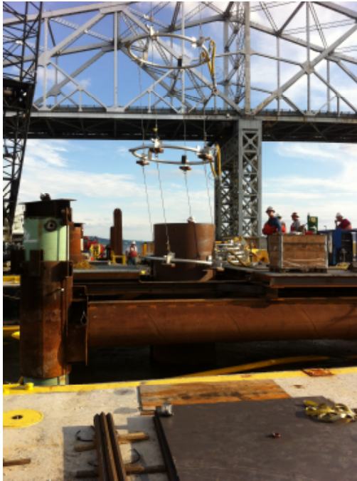
Figure 3. Deployment of the Unconfined Multi-tier Bubble Curtain
