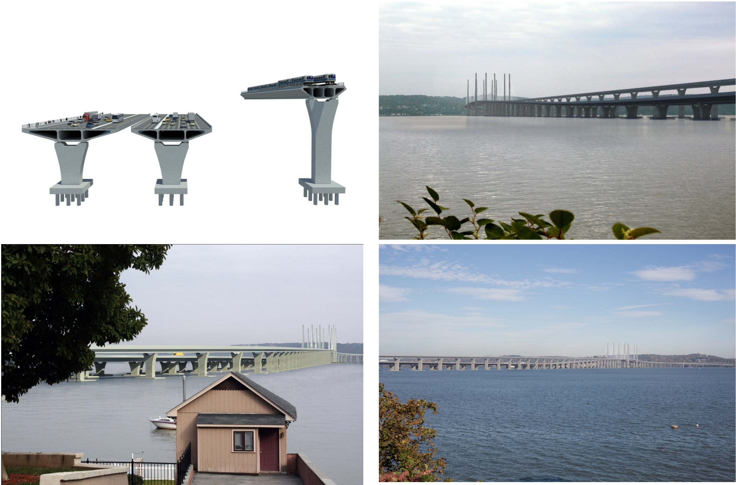
Figure 2.3 – Cross-Section and Visualizations of the Option 2 Rockland Approach with a 3.0% Highway grade and 1.2% CRT grade
