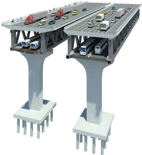
Option 6 – Dual-Level Transit Below Two Structures Two Dual-level structures with highway above and CRT below on the North and BRT Busway below on the South
