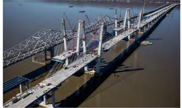
Other innovative equipment includes: TZC's **mobile concrete batch plants**, which supply the majority of the structure's concrete directly on the river; the **self-climbing jump forms** that rose along with construction efforts to create the iconic main span towers; the **protective bubble curtains** used to absorb the energy produced during pile driving; and the **synchronized jacks** used to lower football-field-length foundations into the Hudson River.
