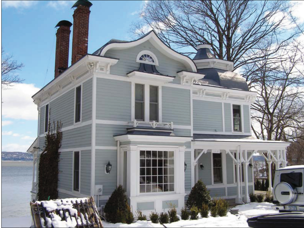
Photo 1. Looking east toward west façade of 147 Piermont Avenue. Note projecting pavilion, wrap-around porch, ogee-shaped roof, interior chimneys with corbelled caps, and historic fenestration pattern.
