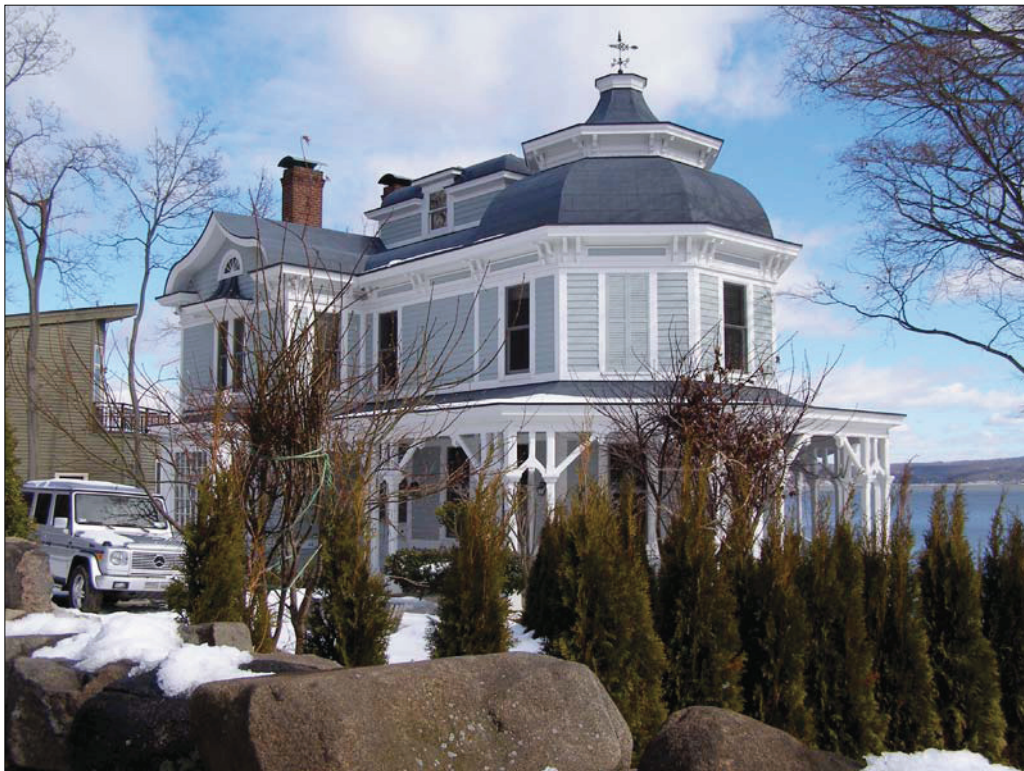
Photo 2. Looking northeast toward 147 Piermont Avenue. Note pentagonal-shaped section surmounted by a cupola. Residence overlooks the Hudson River and retains a high degree of integrity.
