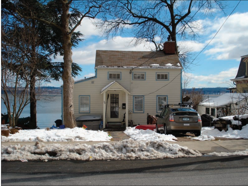
Photo 1. Looking east toward west façade of 129 Piermont Avenue. Note six-over-six double-hung sash and glass-and-panel door on first story, and three-pane frieze-band windows at top half-story, typical details associated with early-19th century workers houses.
