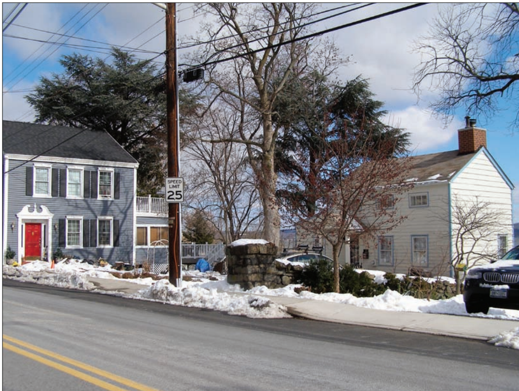
Photo 2. Looking northeast toward south and west facades of 129 Piermont Avenue. Note mature trees which surround residence and contribute to its historic feeling.
