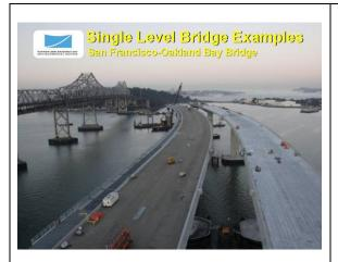
Of interest to note is that this bridge was designed to accommodate rail in the future as a replacement for one lane and one shoulder in each direction.
