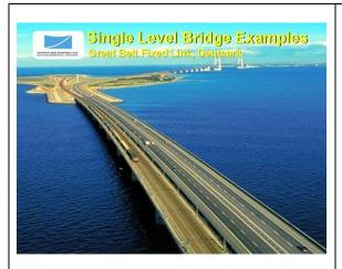
This bridge in Denmark consists of 2 separate bridges, a four-lane roadway structure and a railroad structure.
