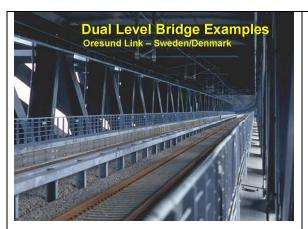
Rail on this bridge is on the lower level. This is the most common method of incorporating rail in conjunction with highway lanes. This arrangement results in symmetrical loads on the bridge structure resulting in the most efficient design.
