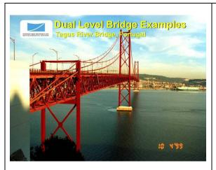
The Tagus River Bridge in Portugal was built as a two level bridge with highway on top and an allowance for rail on the lower level in the future. When the rail was added below the roadway, a second set of main suspension cables was also added carry the increased loads.
