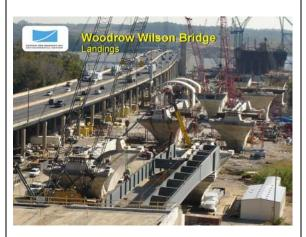
This slide shows the construction of the Woodrow Wilson Bridge at one of the landings. The image shows the existing highway in operation and construction of the full width of the replacement bridge.
