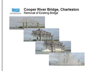
This slide shows the explosive demolition method used for removal of the Main Spans of the old Cooper River Bridge. This type of demolition is unlikely for the TZB because of the resulting impacts to the river and possible impacts to aquatic life.
