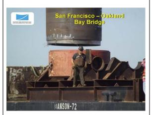
This image gives a good impression of the size of the foundation pile. The construction worker stands beside an 8-feet diameter section.
