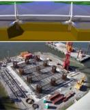
These pictures show the bridge's foundation construction for the Cooper River Bridge. All the images show the construction of the foundations for the diamond towers.
