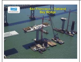
This image, the second of four construction sequence images shows the construction of a pie above the pilecap. For the SFOBB the piers were concrete and were cast-in-place. In many other modern bridges pre-fabrication of the piers offsite is used to limit the period of construction on site and possible environmental impacts.
